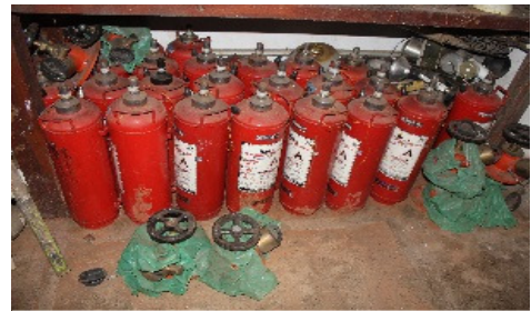
Fire extinguishers lying without installation
